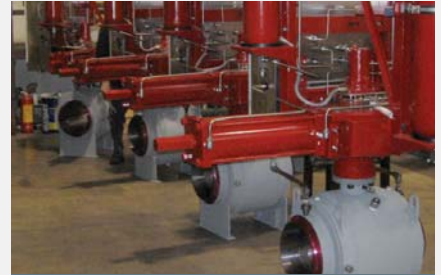
12" 150 Fully Welded Body
