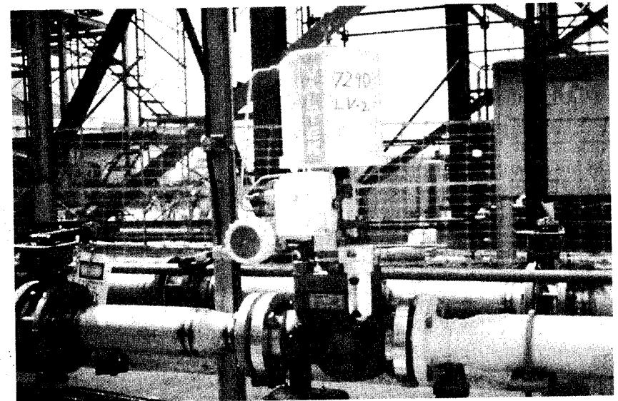
Figure 7.12. Piston cylinder actuator. (Courtesy of Valtek International)
